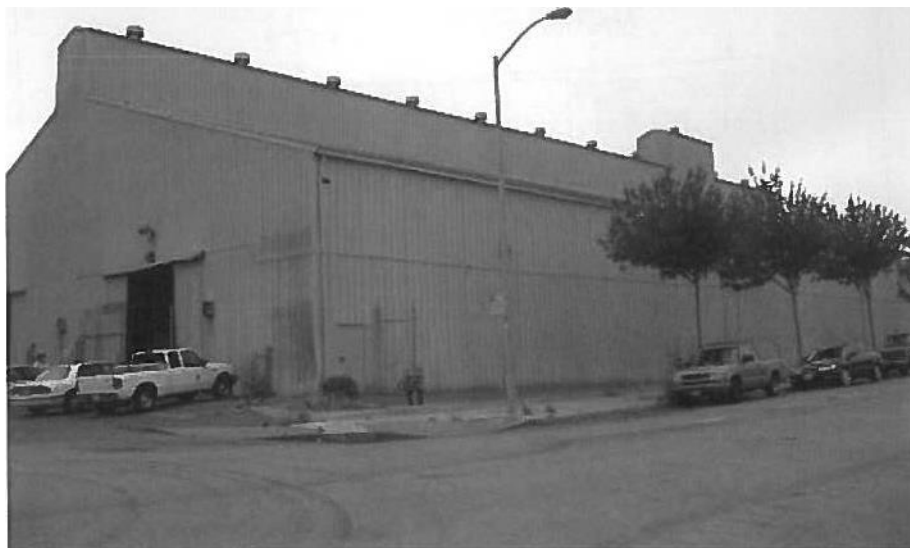
Photograph #10 -View looking southeast
