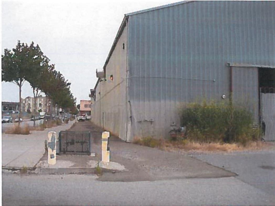
Photograph #1-Exterior view
