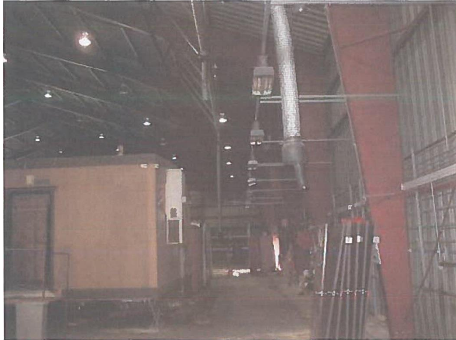
Photograph #3 -View of column
