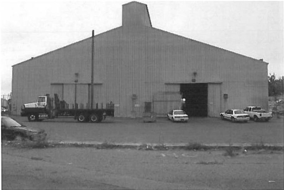
Photograph #7 -View looking south
