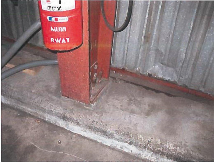
Photograph #5 -View of foundation
