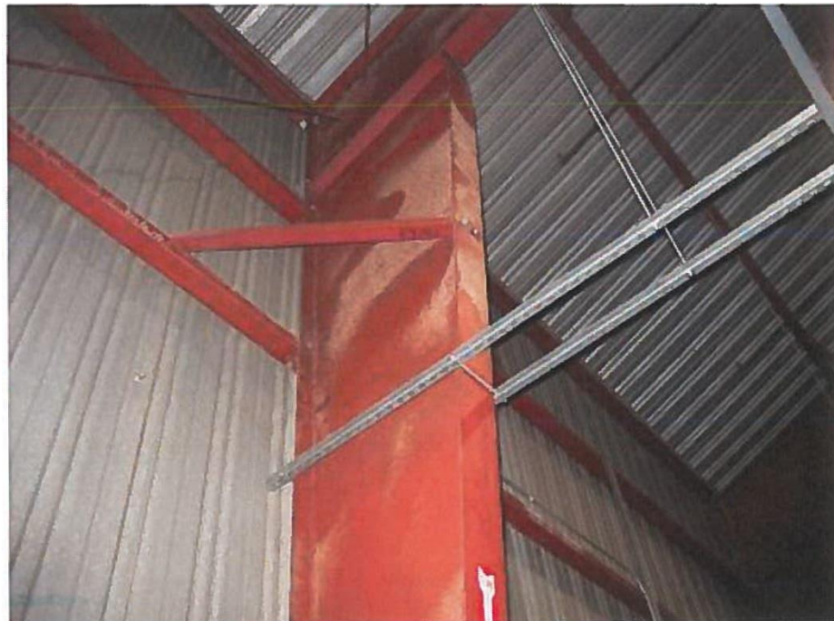
Photograph #4 -View of column looking upward
