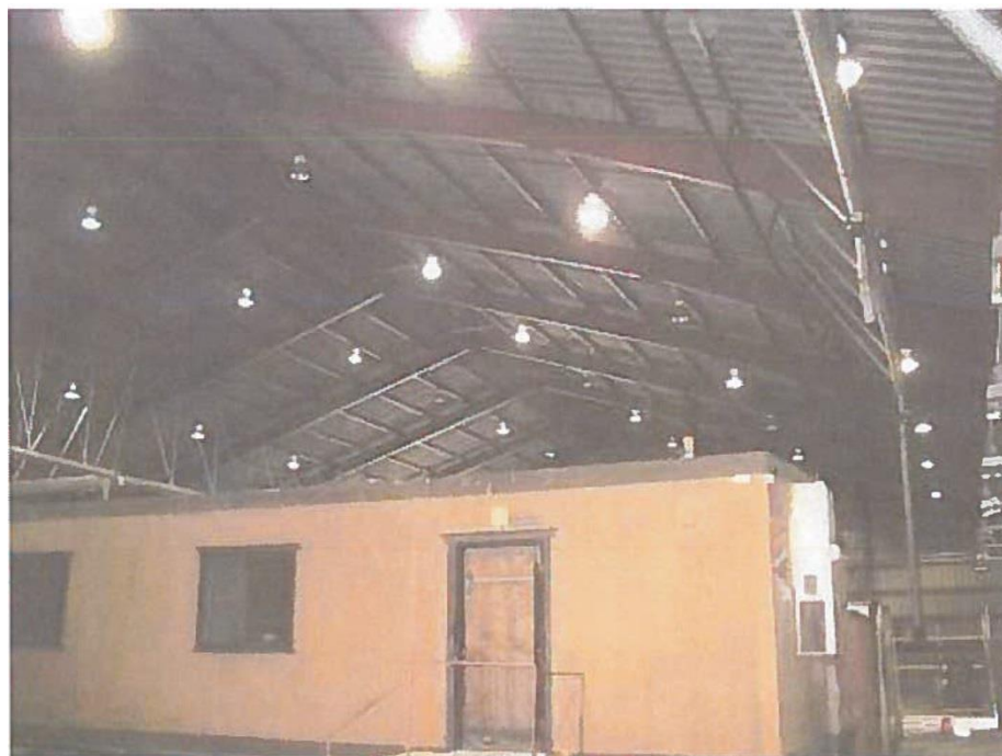
Photograph #2 -Interior view of framing
