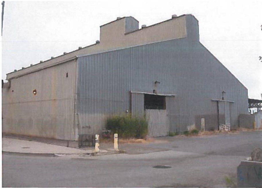
Photograph #11-View looking northeast
