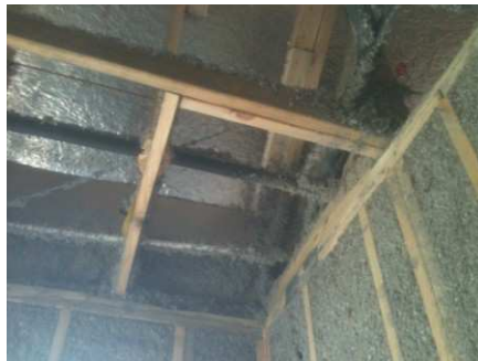
Dead wood needed in master bath closet
