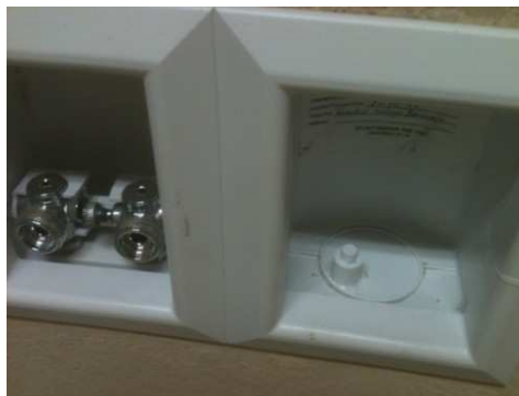
Drain plug as washer/drain box to be removed
