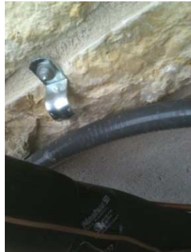
AC conduit no longer strapped (2 locations) Outlet cover above frig cabinets doesn't cover opening
