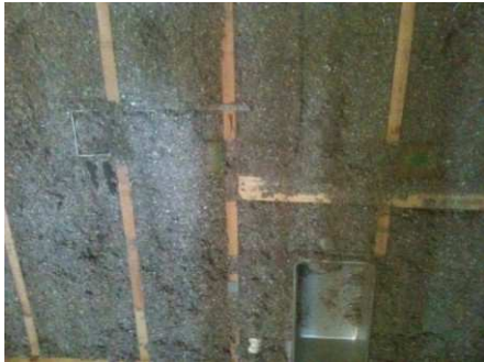
Laundry room wall
