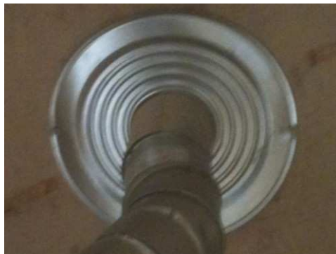
Draft stop could use two more screws for better seal
