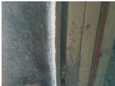
Warped return at breakfast window (OSB)
