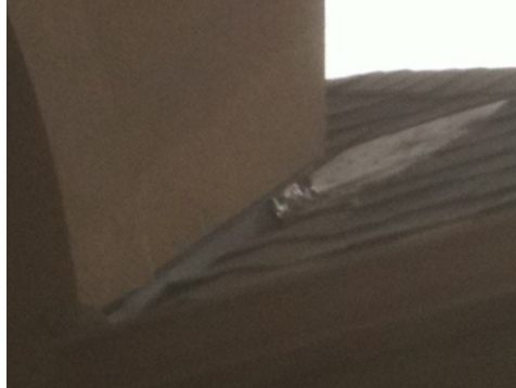
Tape or other foreign object in run-off path at roof
