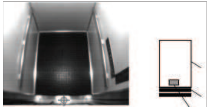
Figure 5: Correct mounting location for ESPROS/VOL-A on wall of elevator cab above elevator door
