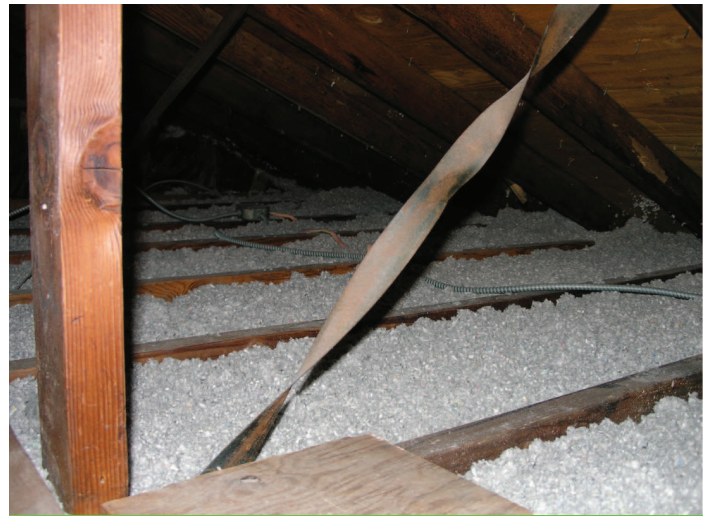
Blown cellulose insulation in attic
