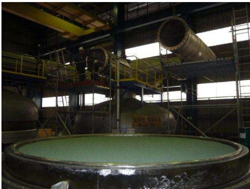
Figure 2: Installation of secondary catalyst
