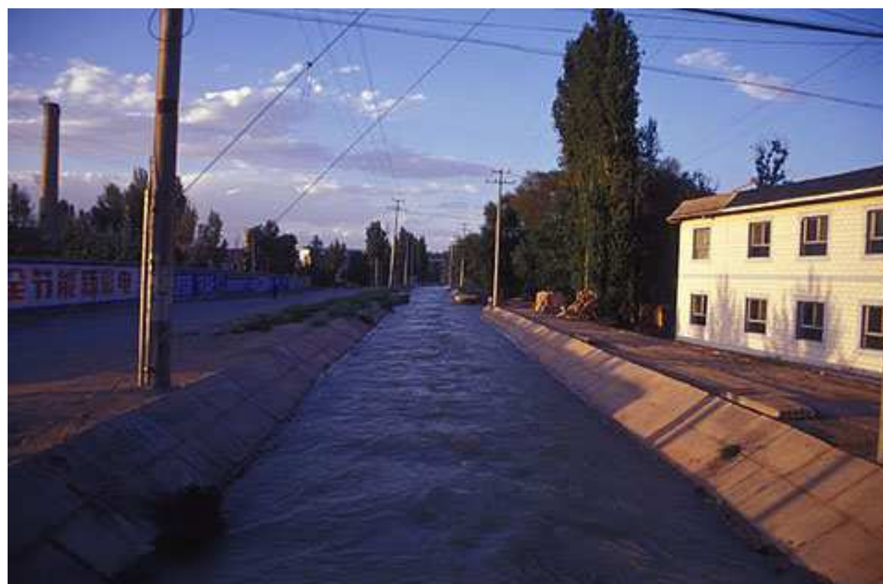
Open-air channels used to distribute water throughout the Hexi corridor are subject to rapid evaporation, day in and day out.
