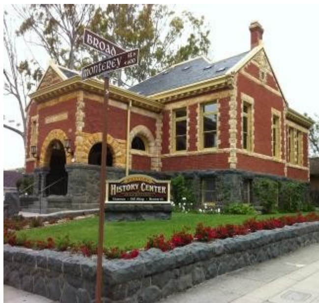
San Luis Obispo County History Center and Museum. It began as a Carnegie Library in 1905, and was built of brick, yellow sandstone, and blue granite. Photo: Jacqueline Williams.
