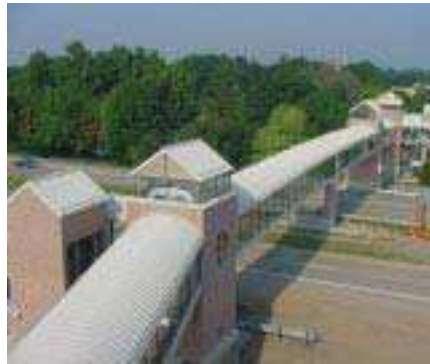
This unique design utilized a double-layered free-span system eliminating intermediate framing while also providing an insulated system for a climate controlled canopy.
