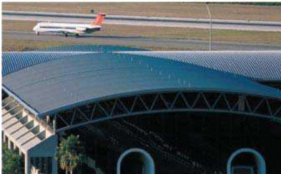
Zip-Rib applied to intersecting barrel vaults. Gentle radius results in low slope; thus weather-tight performance of roof panel is critical.
