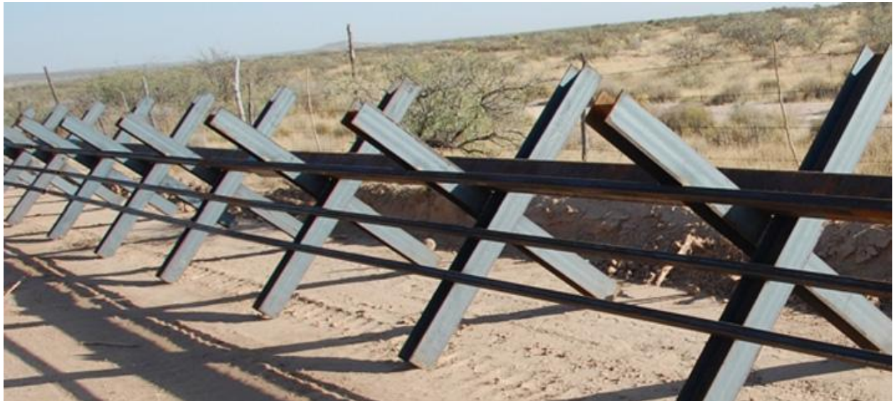
FIGURE 1 SAMPLE IMAGE OF BARRIER STYLE, SIMILAR IN DESIGN TO THE PROPOSED PROJECT
