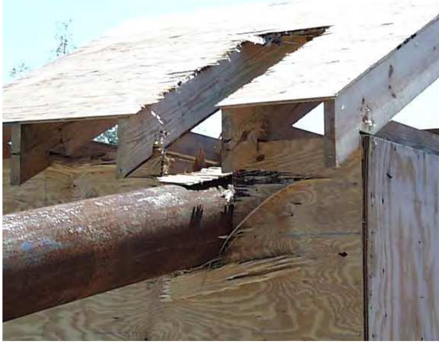
Figure 12.27. Large Pipe Impacting Roof and Wall With Plywood Sheathing, 7600 lb-ft at Impact, Breaking Roof, Top Plates and 1/8 Wall.
