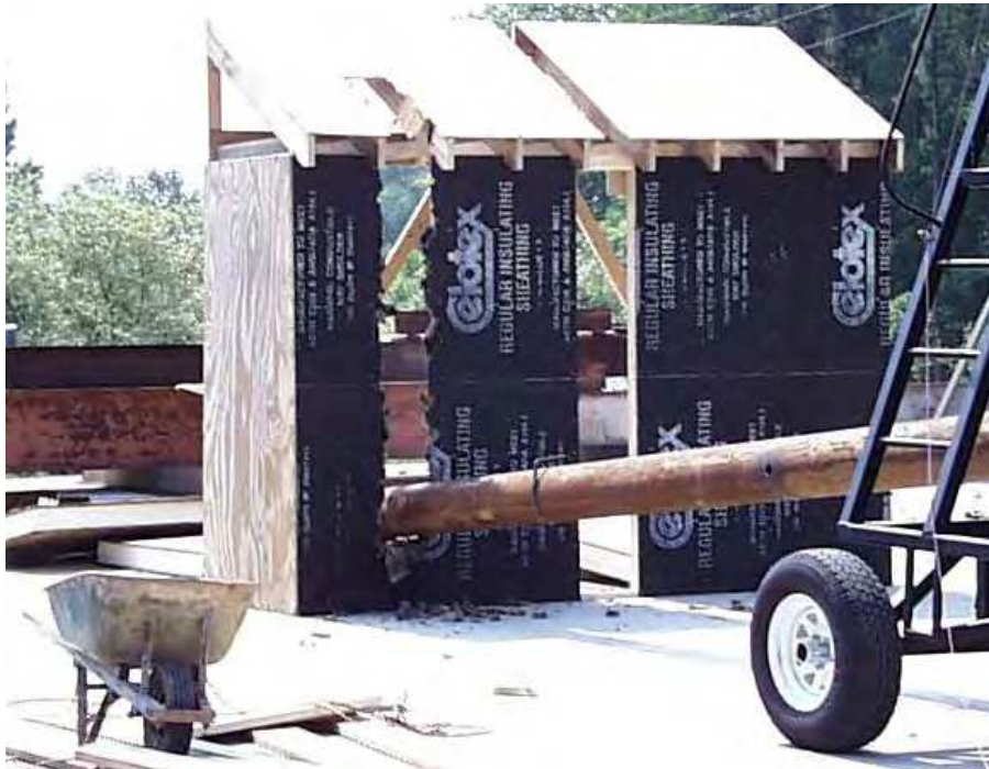
Figure 12.26. Large Pipe Impacting Roof and Wall Without Plywood Sheathing, 7600 lb-ft at Impact, Breaking Roof, Top Plates and Entire Wall with Apparent Residual Energy Hitting Ground.
