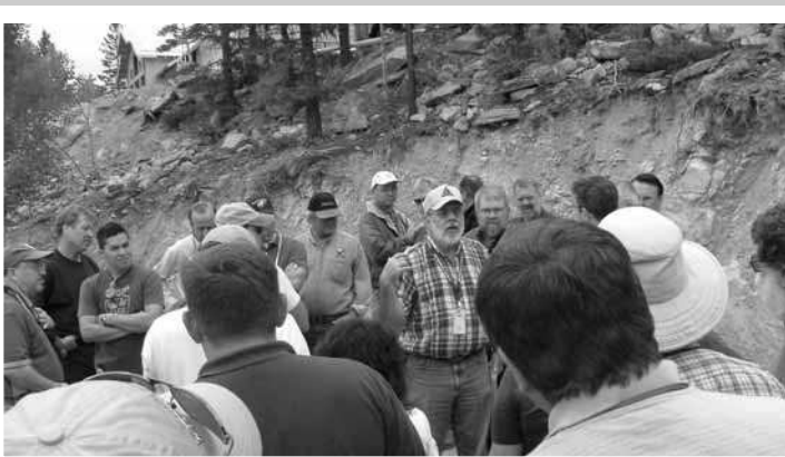
Field trip participants visit a residential onsite installation site outside of Denver. The field trip provided hands-on installation experience and participants were able to speak with local regulators, manufacturers, and installers.
