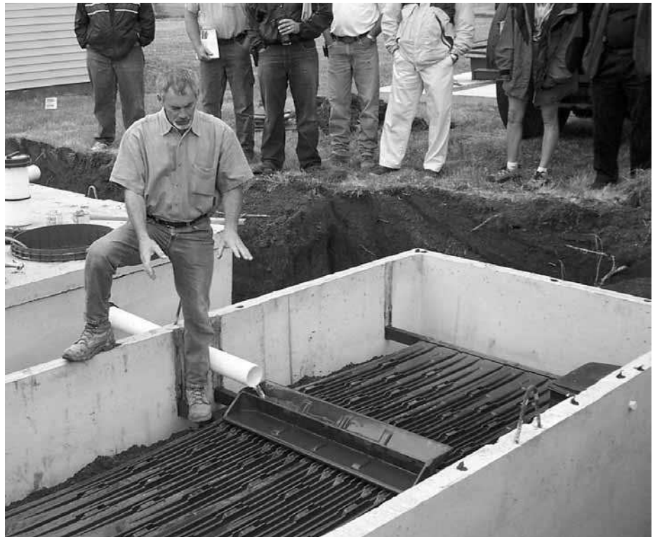
Bob McKinney, president of River to River Onsite Septic Solutions in Waukee, IA, and past president of IOWWA, explaining how the peat system works.
