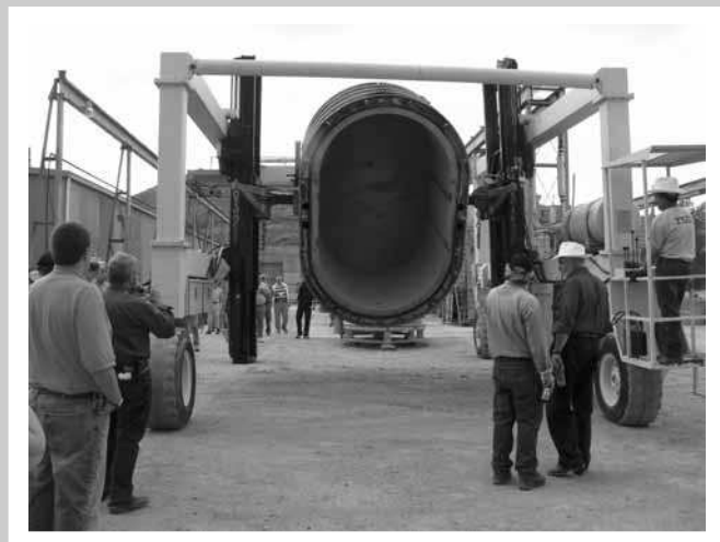
Front Range Precast Concrete president, Doug Jatcko , shows field trip participants the Halo direct control robot that allows a single operator to manipulate forms, strip tanks, move inventory, and load trucks efficiently and safely. This greatly reduces necessary manpower, increases levels of quality assurance and control, and allows precast concrete manufacturers to effectively concentrate on mass production.
