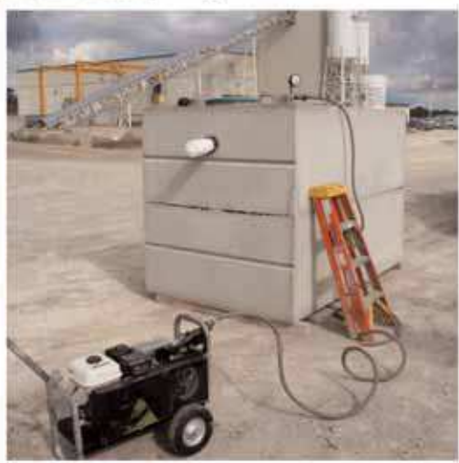
Testing at the plant.
