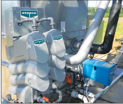
Closed Circuit Cooler Baton Rouge, LA USA
