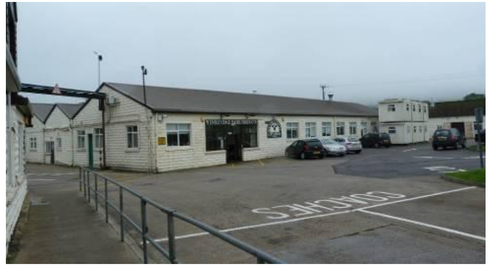
The existing Cheese Production facility
