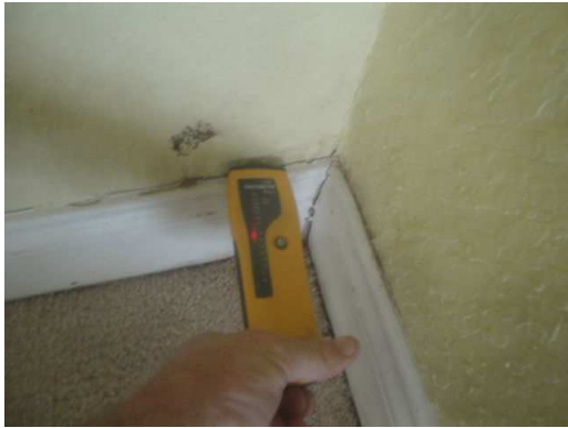
water intrusion/mold
