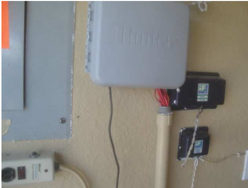
conduit loose at control panel and wall
