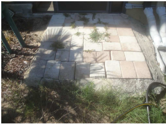
brick pavers settling
