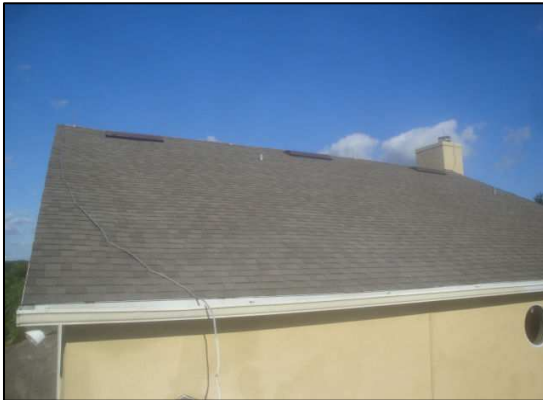
shingles in fair condition
