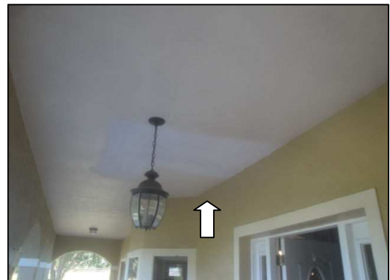
ceiling damage on front porch requiring repair/finish work
