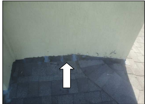
tarred in flashing
