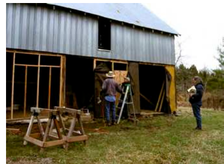
Remodeling portion of barn for equipment and tool storage.
