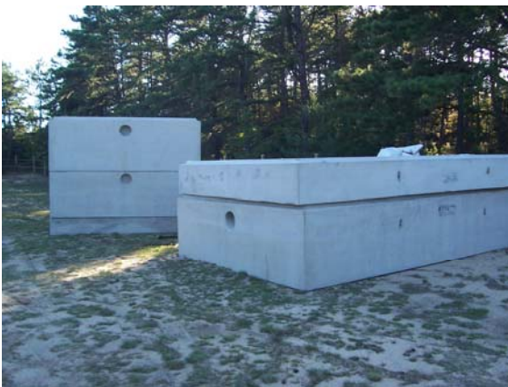
Getting ready to install a 10,000 GALLON SEPTIC SYSTEM
