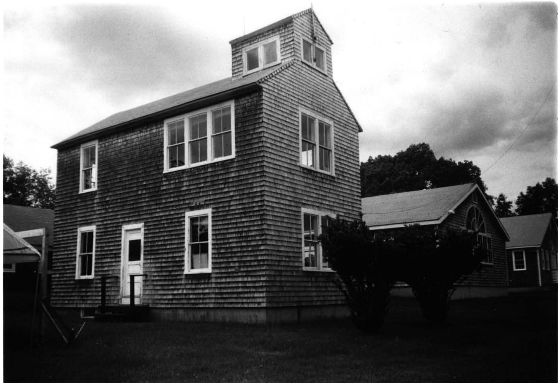
Mavis Wireless Station Kent County, East Greenwich, RI Photo #1 of 2
