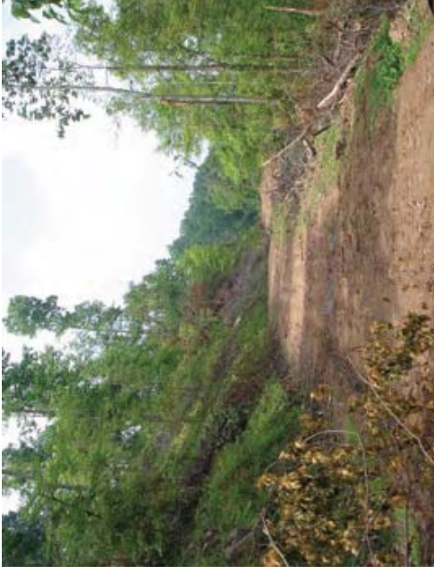
Well-constructed skid road
