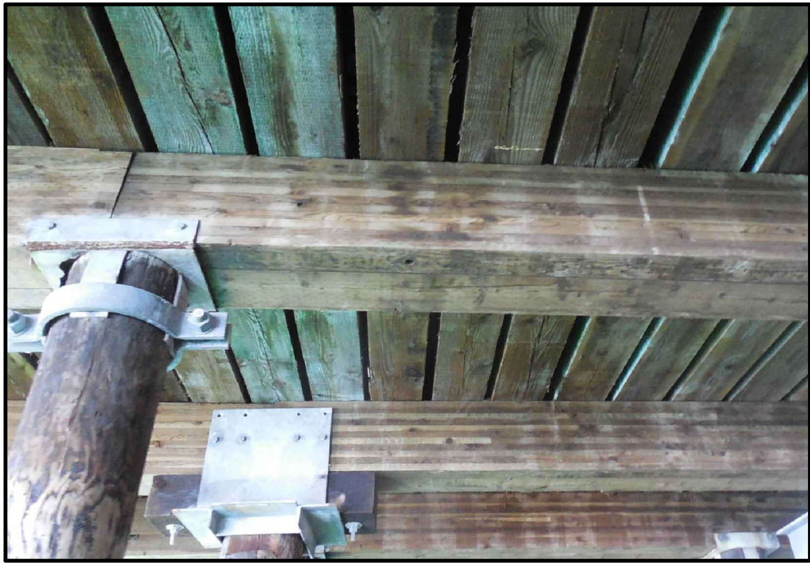
GLULAM PILE CAP AT HEAVY LIFT ZONE
