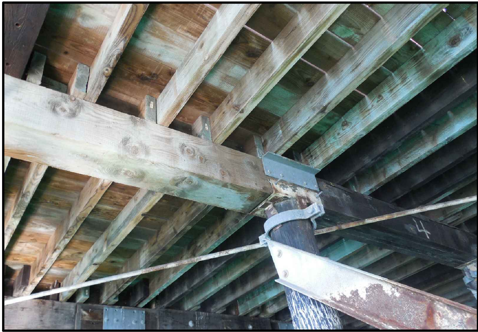
TYPICAL PILE CAP AT WHARF
