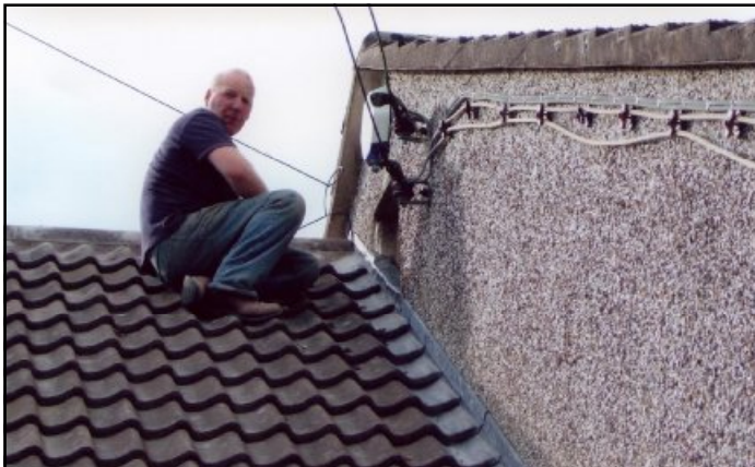
Raymond King completes the roof on the hall extension.
