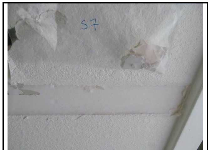
Photograph No. 018: Sample 7 - Drywall joint compound
