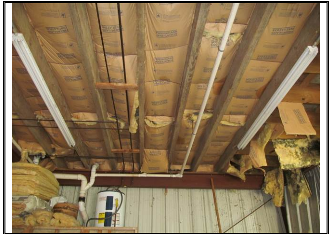
Photograph No. 005: Garage overall
