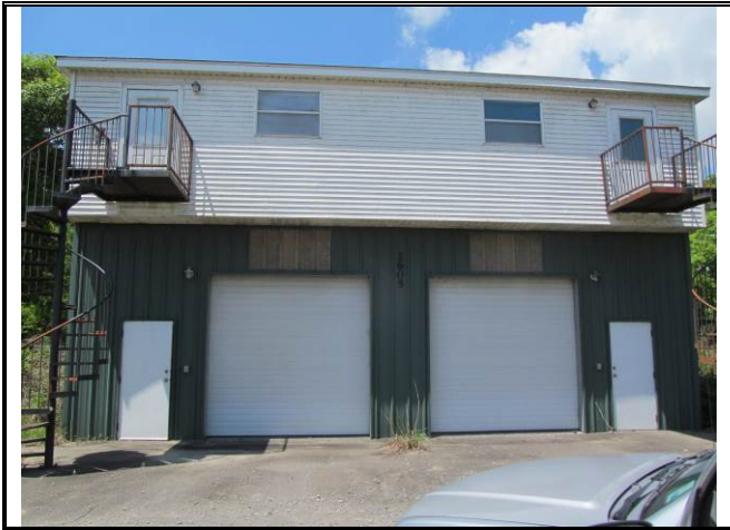
Photograph No. 001: Overall exterior
