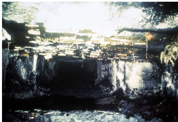
Fig. 5. A degraded scene in underground coal mine.
