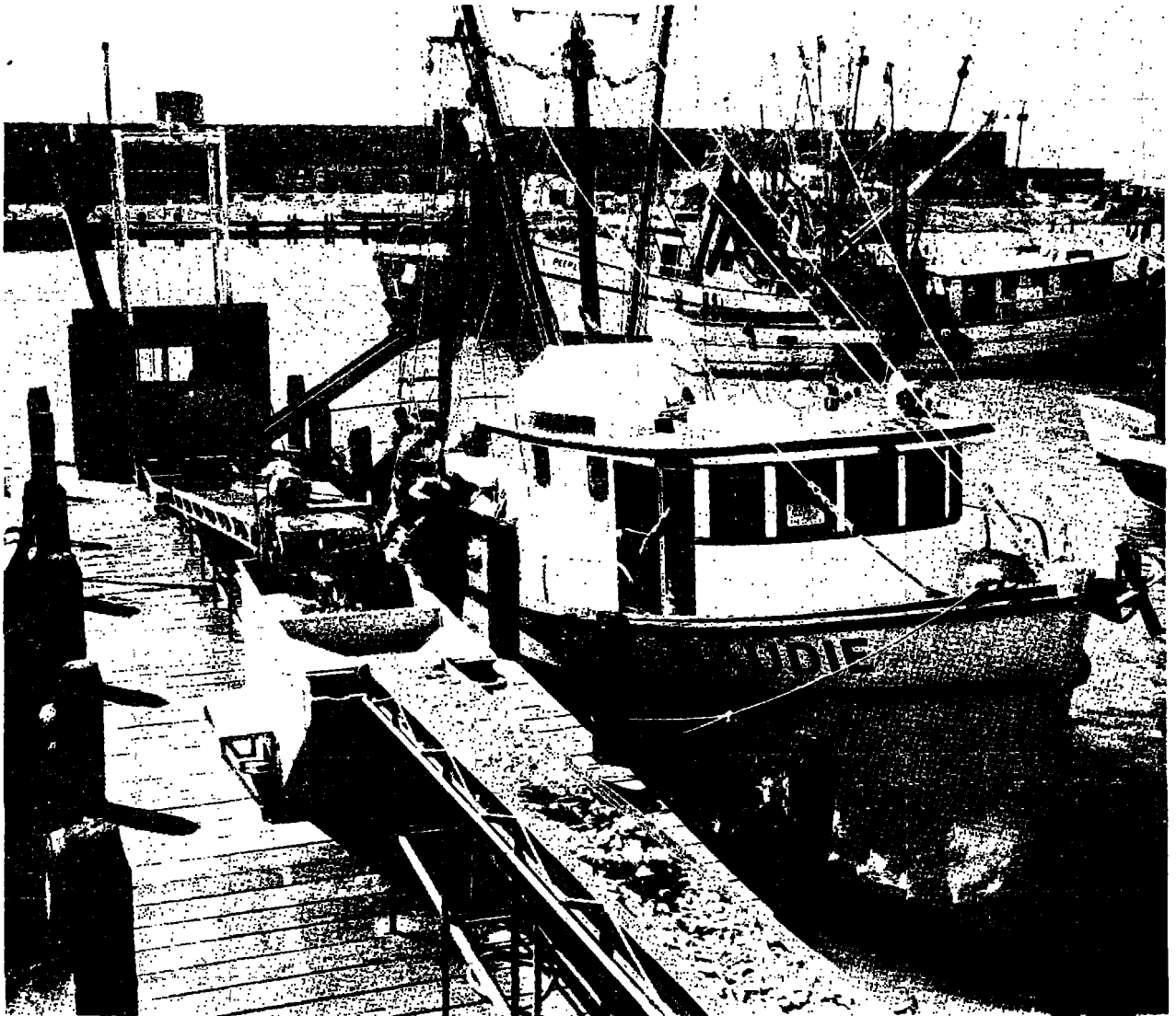
FIGURE 5.—Unloading catch of whole shrimp at a modern Gulf coast processing plant. Hopper (at far end of conveyor) is lowered into vessel's hold and facilitates unloading. (Ice is removed by means of bath situated midway along the conveyor which carries the shrimp to the processing facility.)
