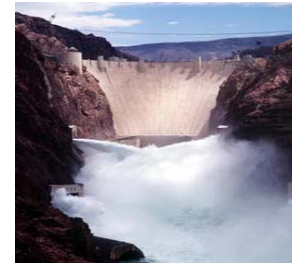
Hoover Dam Boulder City, Nevada
