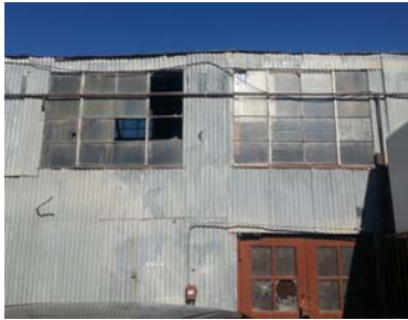
Building Exterior – Broken glass
