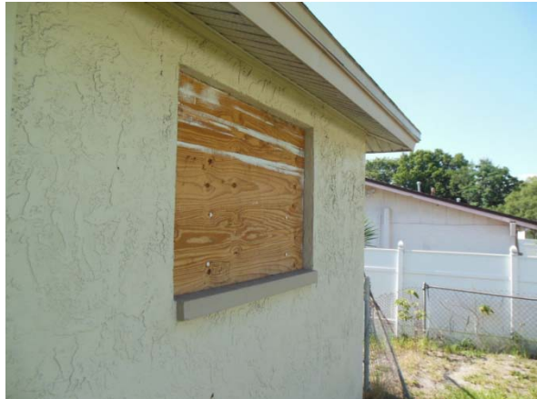
Install new window
