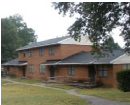
Public housing includes Civic Park, at 72 units, with additional 8 units on Partee St.
