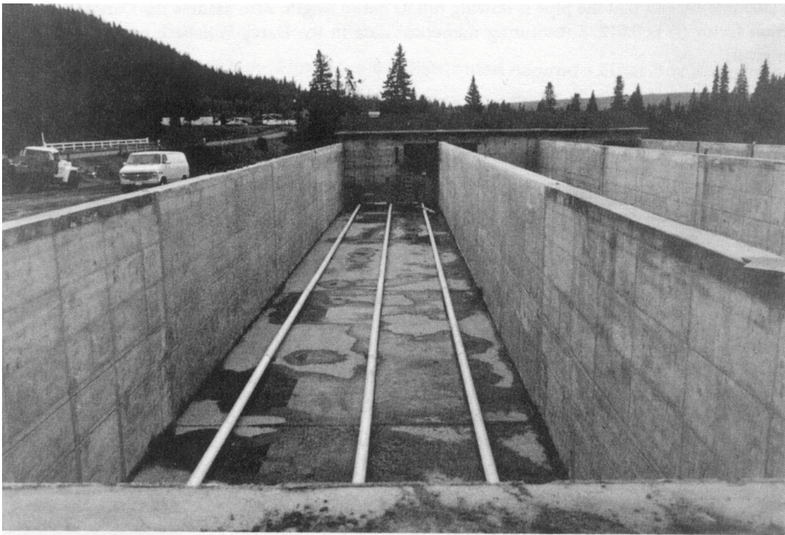
Figure 3-7. Typical Filter Underdrain (AWWA, 1991)
