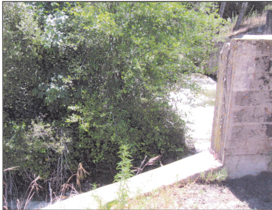
Photo 2: Northeast corner of existing bridge
