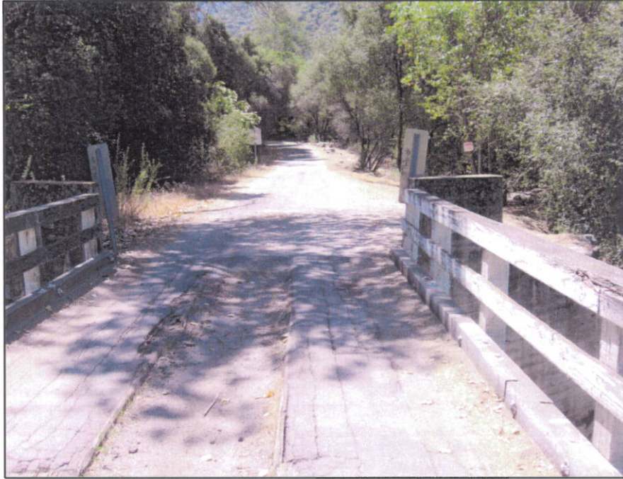
Photo 5: Southern approach to existing bridge
