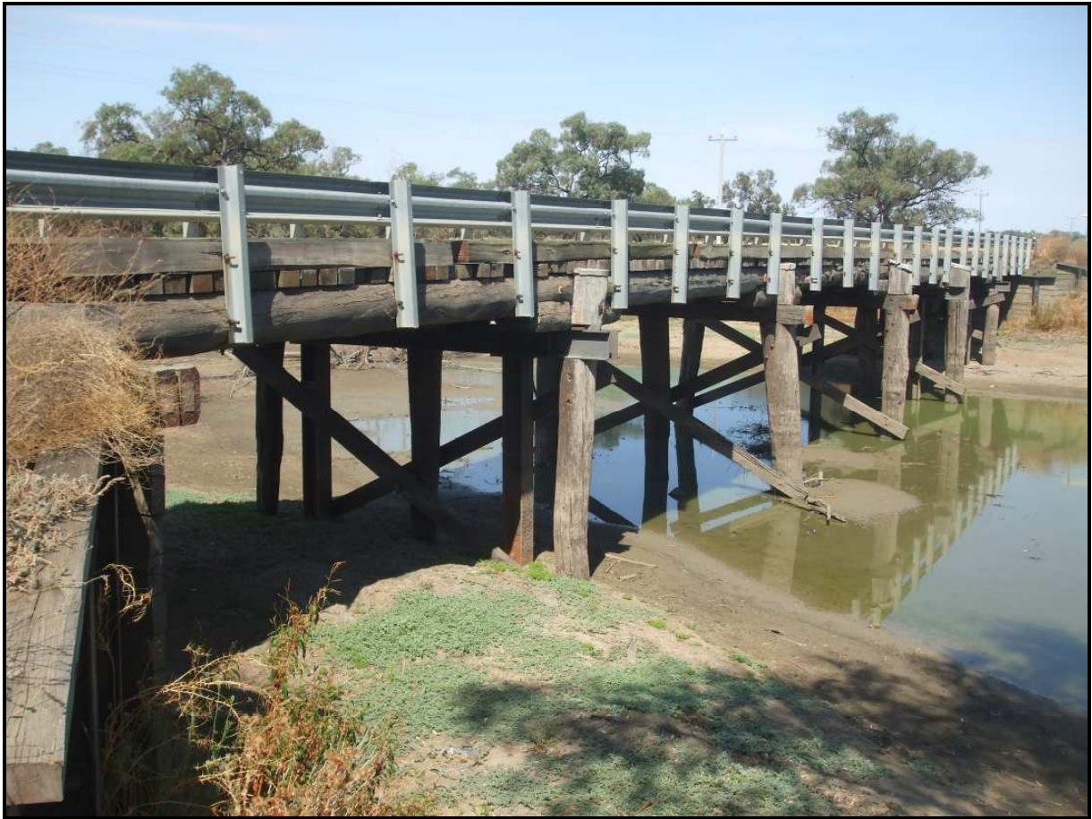
Budgee Creek Bridge – Site Photo Two
