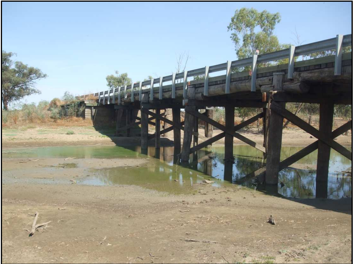
Budgee Creek Bridge – Site Photo One
