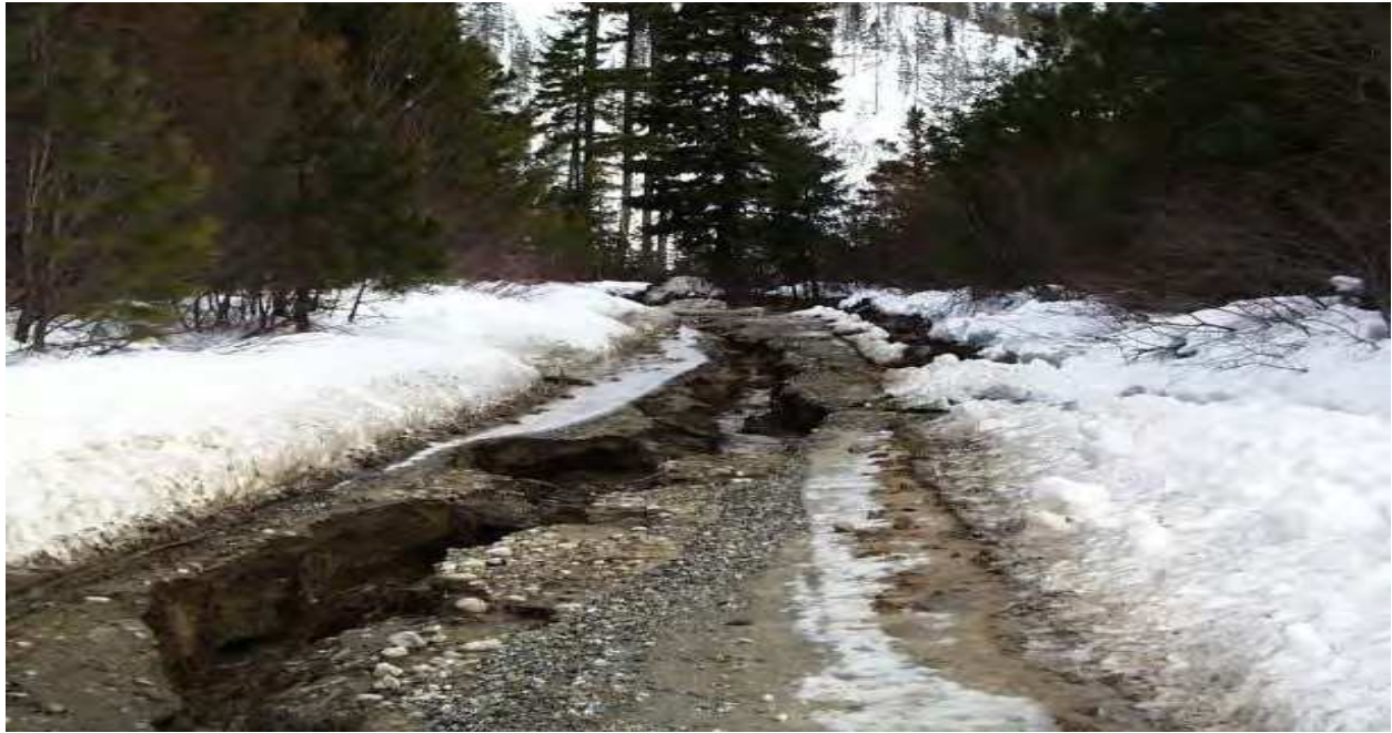
Figure 1: Damage created by a landowner improperly snowplowing Forest Service Road 6910 in the Wenatchee-Okanogan Forest in November, 2008. Photo is courtesy of Forest Service.
