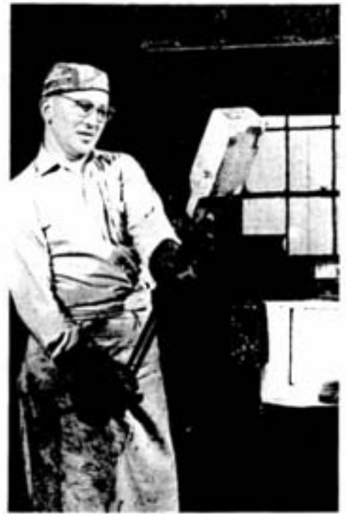
Paul Oleksiw removes a blank from an oil-fired forge where it is being heated to become a crusher wedge for the Copper Cliff casting building.
