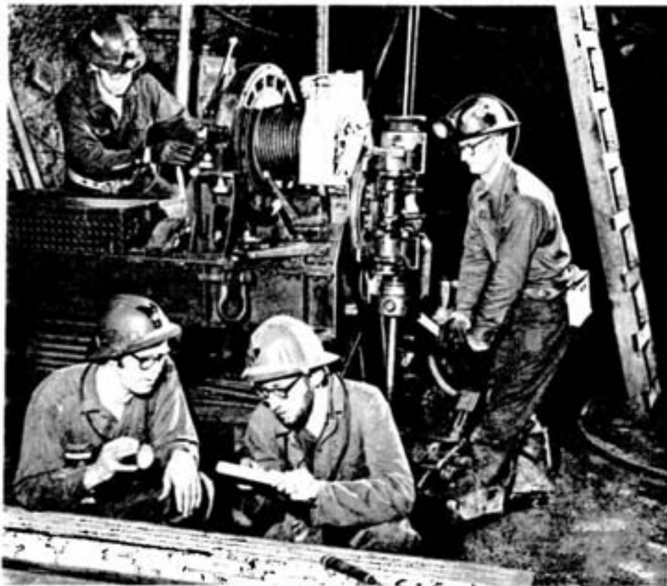
Although South mine has been in operation for about a year, development is continuing to define the future potential of the ore body. This diamond drill is set up on 2000 level where mine geologist Don Brown is discussing some of the core samples with drill foreman Charlie Kirby. In the background, Rudy Jolicoeur greases the drill for operator Val Gionet.
