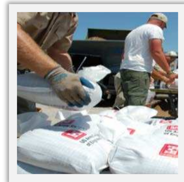
Sandbags to prevent intrusion of water
