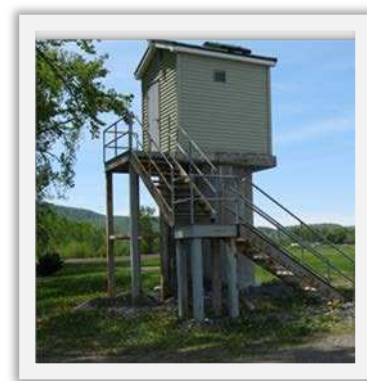
Wellhead above 100-year flood
