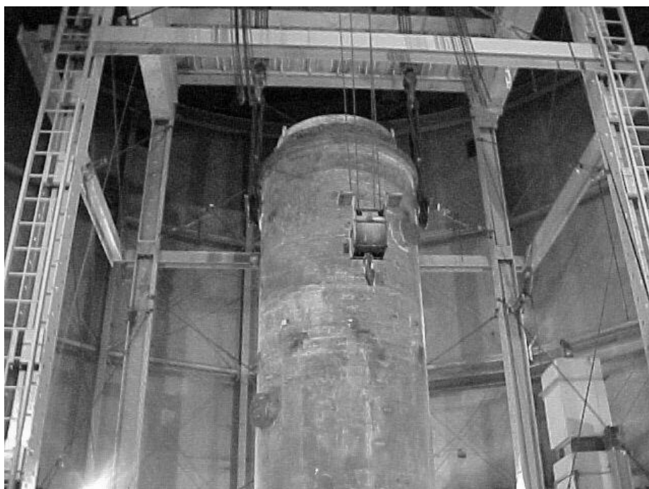
FIGURE 2.1 Lifting the Tank with the 600 Ton Jacking Tower
