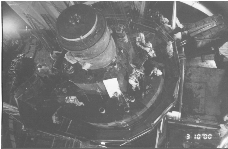
FIGURE 2.2 Removing the Biological Shield
