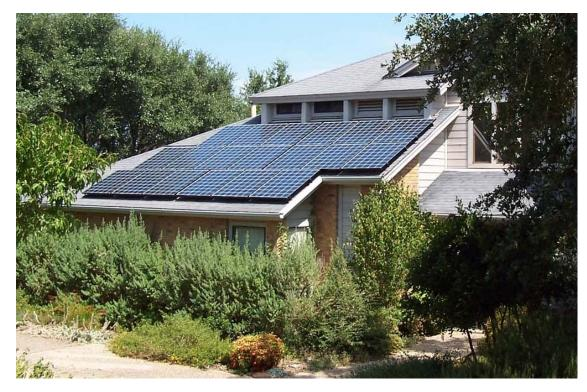
This is an example of a 3kw system consisting of 18 panels @ 175 watt each.
