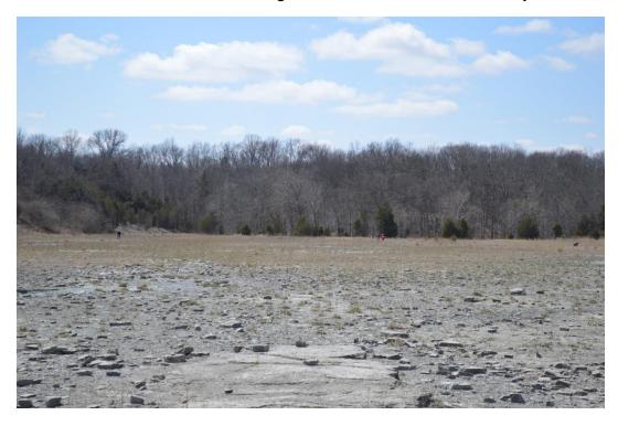
Typical view of the broad, flat emergency spillway consisting of an exposed limestone bed surface littered with complete and fragmented Ordovician fossils.
