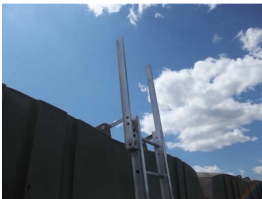
Bolt the ladder into the lifting lug.
