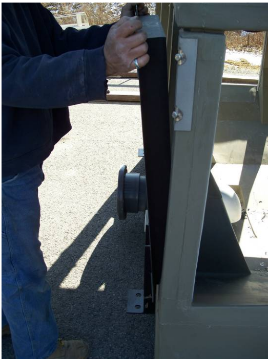
Set the louver in the opening.
