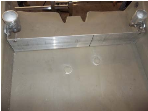
The kick-plate will be away from the ladder. Handrail fittings are already installed in place on the cooling tower. The handrail fitting has a set screw for securing the aluminum pipe.
