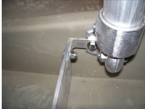
The kick-plate will be away from the ladder. Handrail fittings are already installed in place on the cooling tower. The handrail fitting has a set screw for securing the aluminum pipe.
