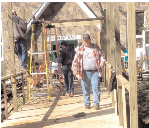
The men work to enlarge the bridge to Hylbert Hall.
