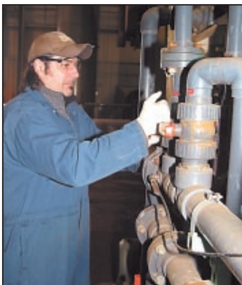
George Natseos opens the valve to release treated waste water at the Everett site.
