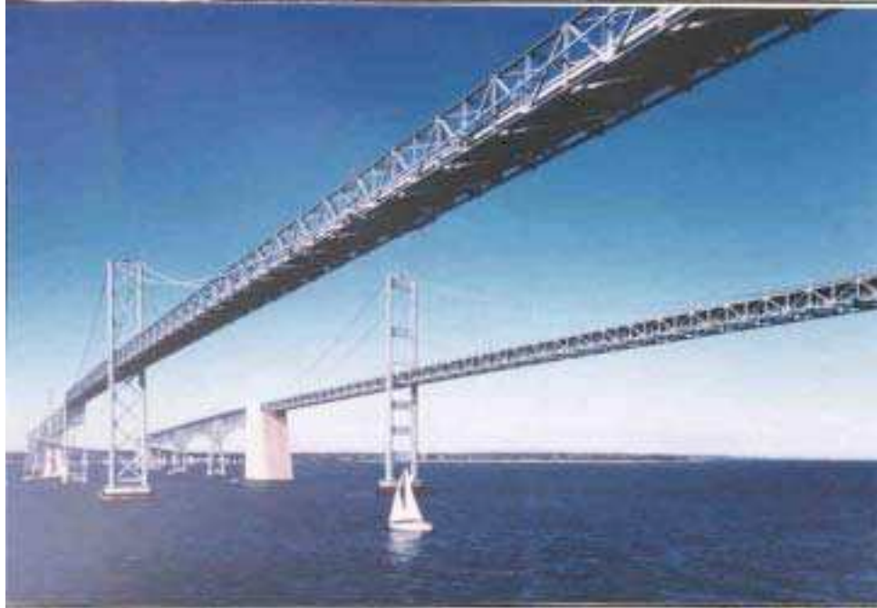
Figure 27. Chesapeake Bay Bridges, Annapolis, MD
