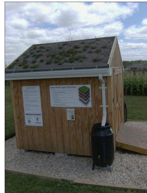
New garden shed at the Ag Center showing two different stormwater BMPs, the green roof and a rain barrel.
