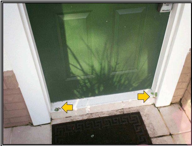
Miscellaneous photo of the live plants at the front entry near the decay damaged wood.
