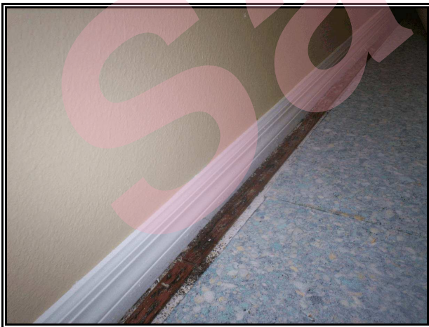
Miscellaneous photo of the water stained carpet tack strip at the front of the dining room.
