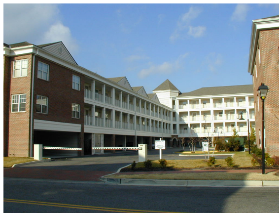
The Heritage at Freemason Harbour.
