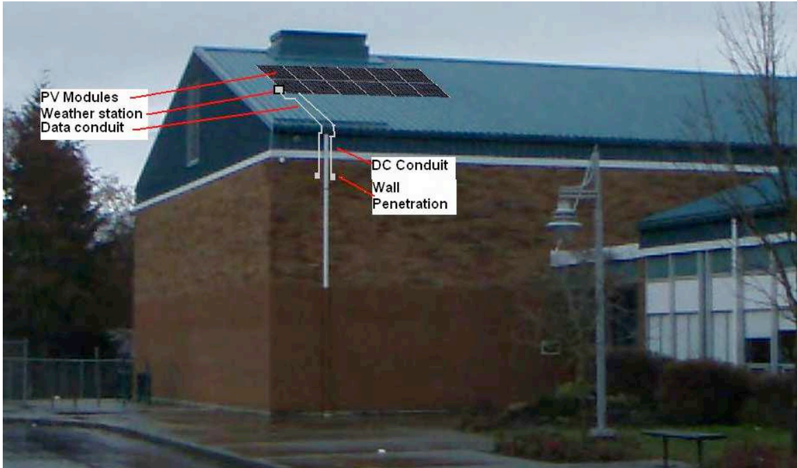
Photo Mock-up of PV array on roof of cafeteria and DC and data conduit running down roof and penetrating wall into backstage area
