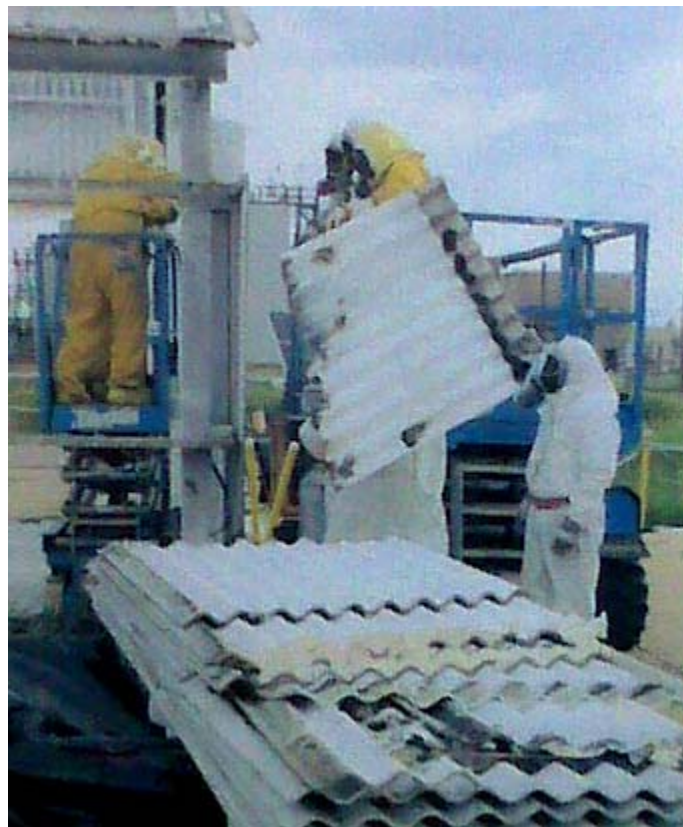
Figure A.5. Transite Siding Removal and Packaging
