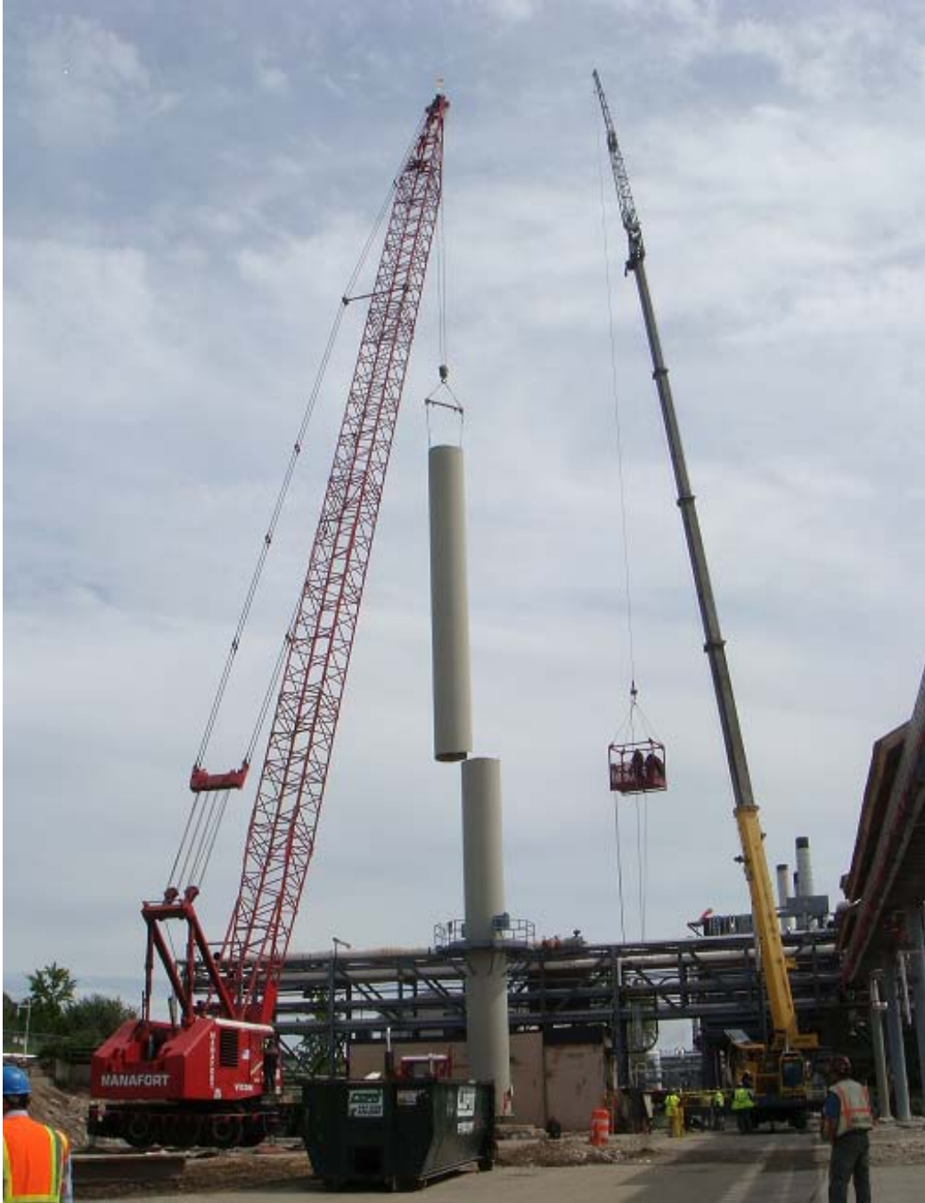
Figure A.11. Stack Demolition (Crane Assisted and OSHA Basket)
