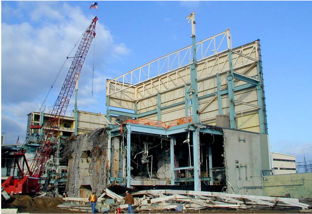
Figure A.8. High Bay Roof Truss Removal (Crane Assisted Disassembly)
