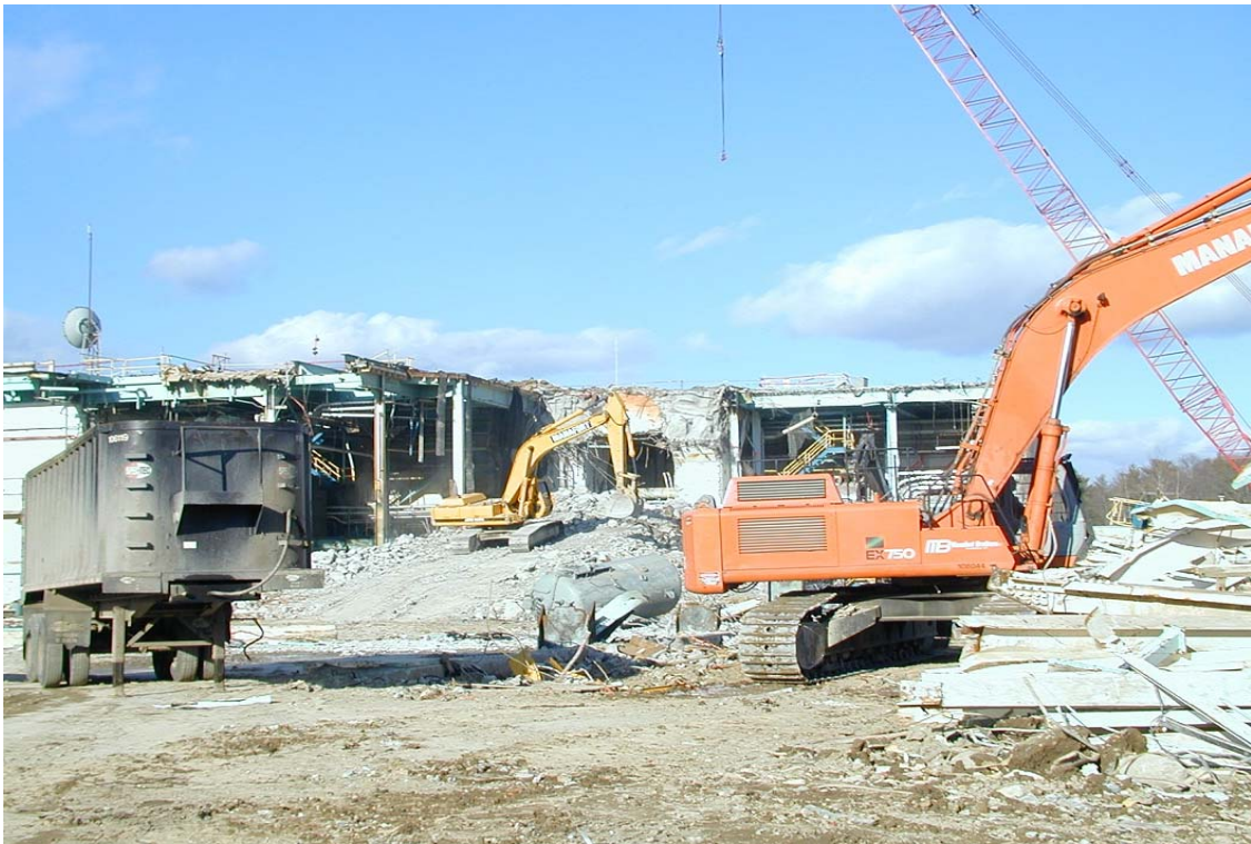
Figure A.9. High Bay Roof Trusses and Columns Removed
