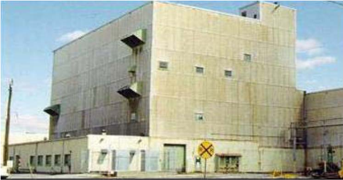
Figure 2. Exterior of the C-410 Complex
