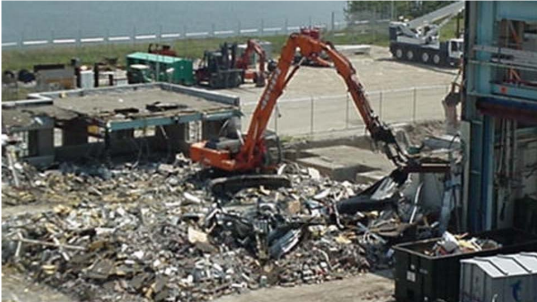
Figure A.6. Building Demolition Using “Long Reach” Excavator with Shear Attachment
