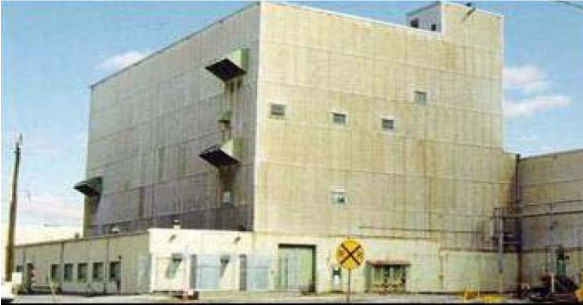
Figure A.2. Exterior of the C-410 Complex
